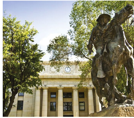
Yavapai Courthouse Plaza
